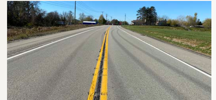
Similar to the completed V10 project immediately north, the Y10 project will include 12 ft. travel lanes and 8 ft. shoulders.
