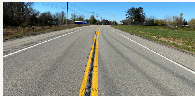
Similar to the completed V10 project immediately north, the V20 project will include 12 ft. travel lanes and 8 ft. shoulders.
